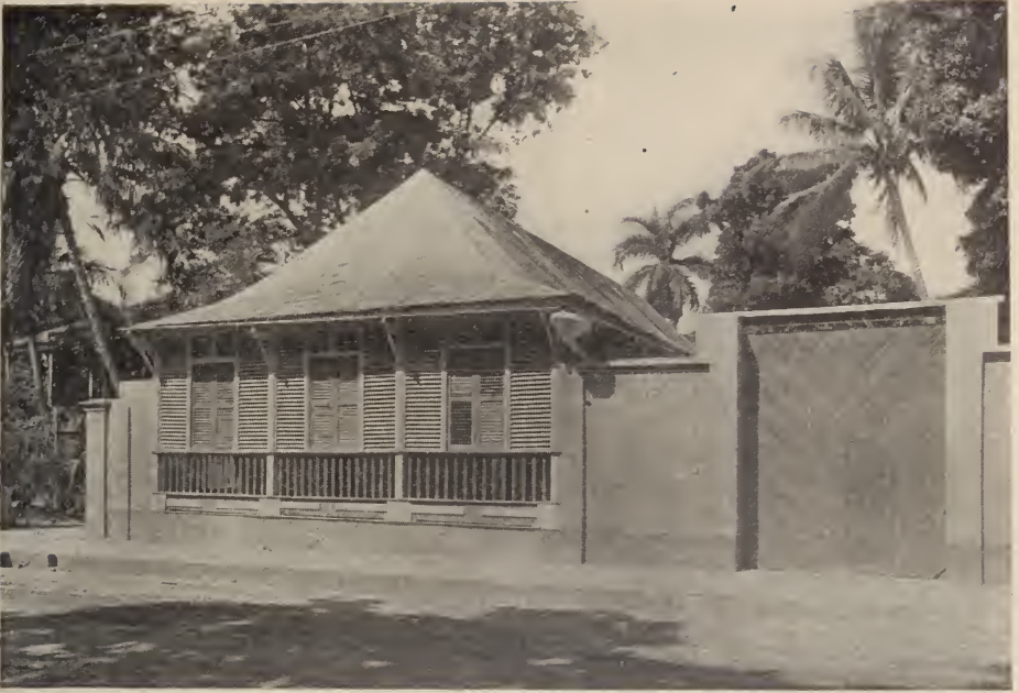
THE EXCHANGE COTTAGE AS SEEN FROM THE STREET
